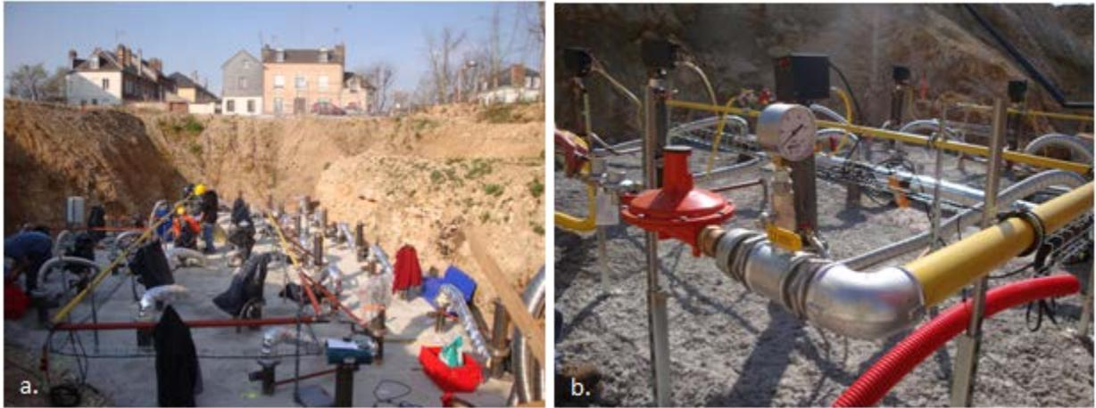
Figure 8. a). Gas distribution system being assembled to feed burners. b). Dual redundant pressure regulators placed in series.
