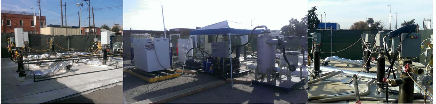
In Situ Thermal Remediation was used to successfully treat benzene, TPH-d, TPH-mo, BaP, and Naphthalene from a former gas plant in EPA Region 9. Gas Thermal Remediation (GTR™), using Thermal Conductive Heating (TCH), raised the temperature of the soils in the treatment zone of the former MGP site to an average temperature of approximately 325 degrees Celsius.
