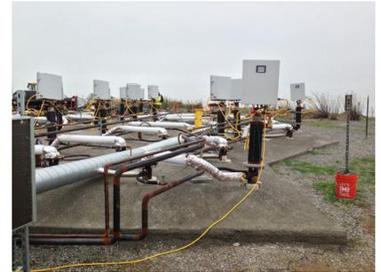
In Situ Thermal Remediation with Gas Thermal Remediation (GTR<sup>®</sup>) is being used to remove NAPL contaminants from a former military base. The system is extracting nearly 1,000 liters of liquid waster every week. LNAPLs, such as fuel and oils, and DNAPLs, such as PCBs and chlorinated solvent, are being removed from the subsurface to make way for a residential homes.
